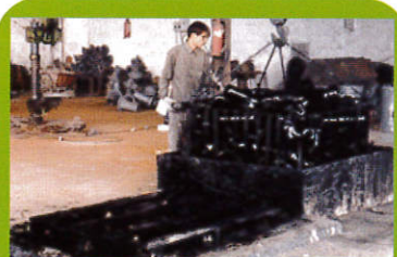
塗瀝青油 Coating Of Bitumen
